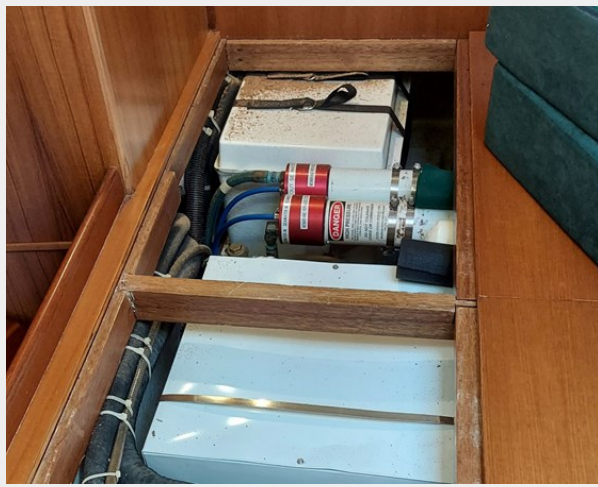
1089 Night Flight Battery box and RO Membranes
