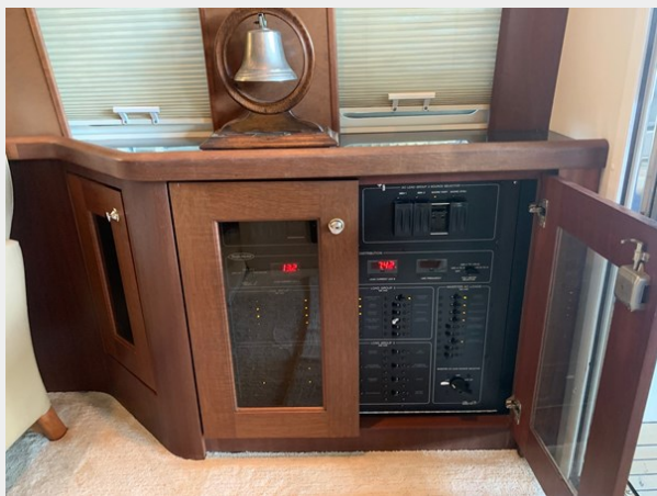
DC Electric Panel
