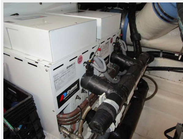
New AC Chillers
