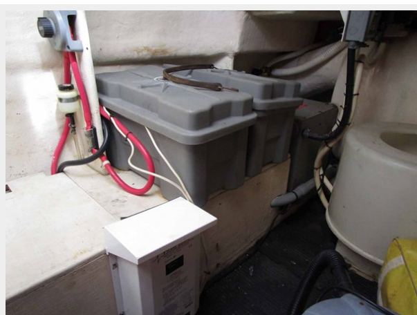
Stern Thruster Batteries
