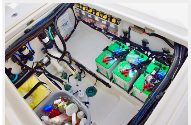
Batteries and equipment under cockpit deck
