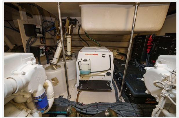
Engine room view 3
