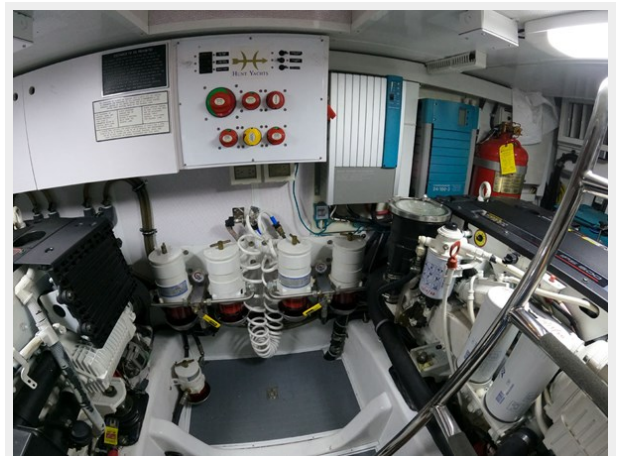
Engine Room Forward Bulkhead
