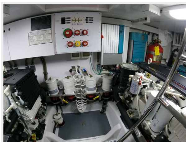
Engine Room Forward Bulkhead
