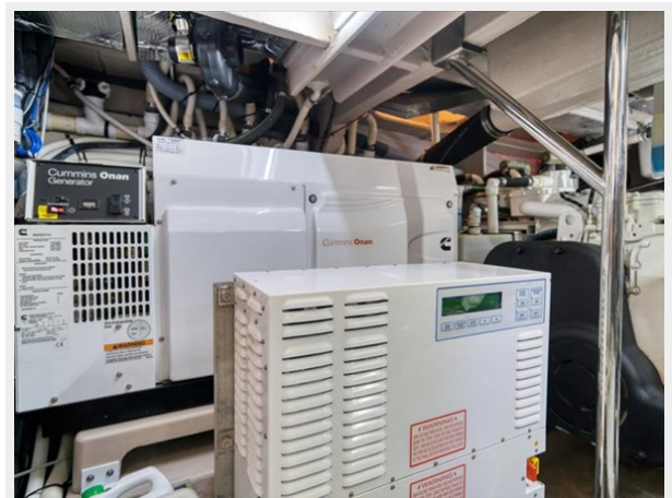
A/Sea Shore Power Converter
