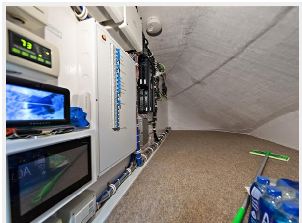
Storage Attic Behind Galley
