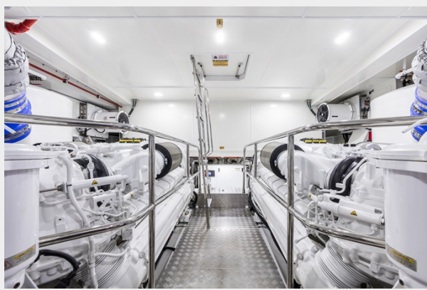
Pearl 95 - Engine room
