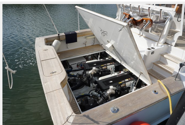
ENGINE ROOM DECK HATCH (003)
