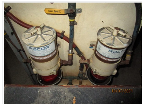
51_2783795_44_thompson_racor_fuel_filters
