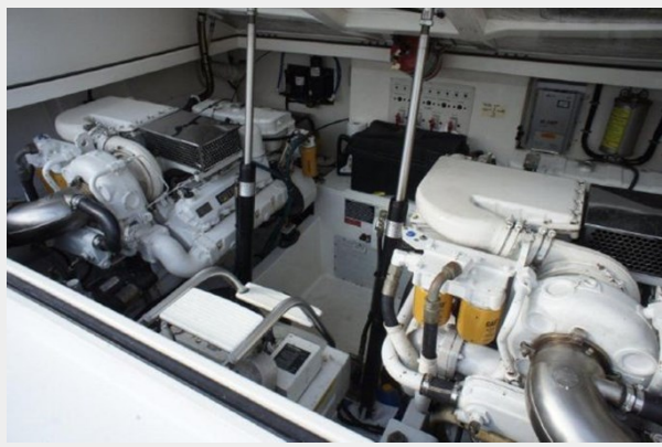
Electric deck lift for engine access
