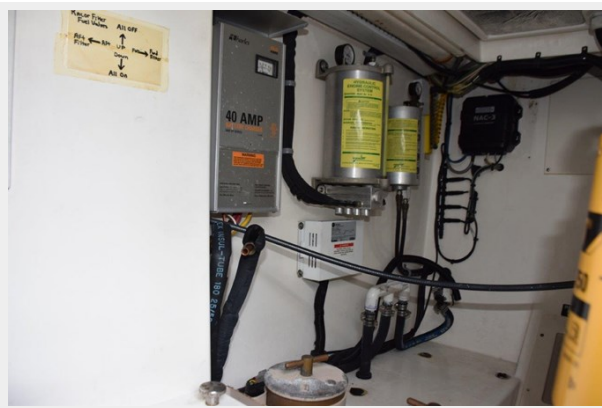
Forward starboard engine room bulkhead
