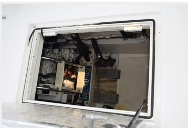
Quick check deck hatch entry to Engine Room
