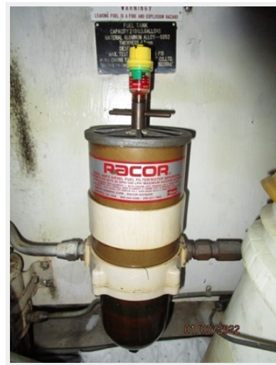
57_2785467_43_jefferson_port_racor_fuel_filter
