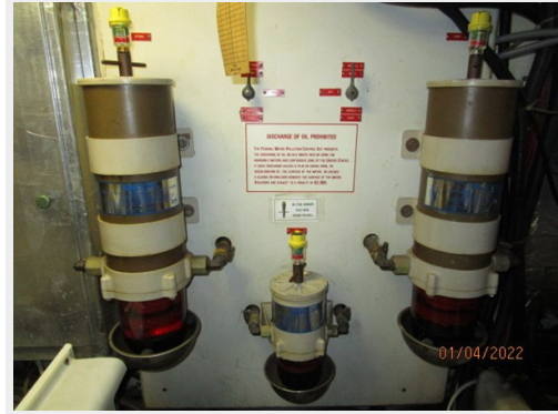
61_2785540_48_californian_racor_fuel_filters
