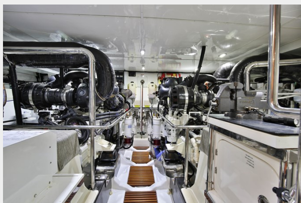
Engine Room facing Aft
