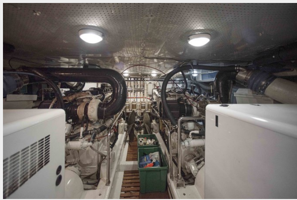
Engine Room Looking Forward
