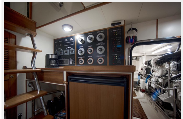
Engine Room Aft Wall
