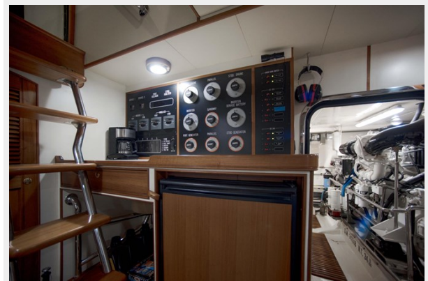
Engine Room Aft Wall
