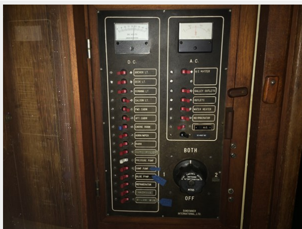
25 Hobo 1984 Sundowner Tug Electrical Panel
