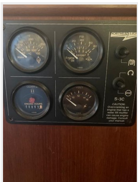
1984 Sundowner Tug 30 generator panel
