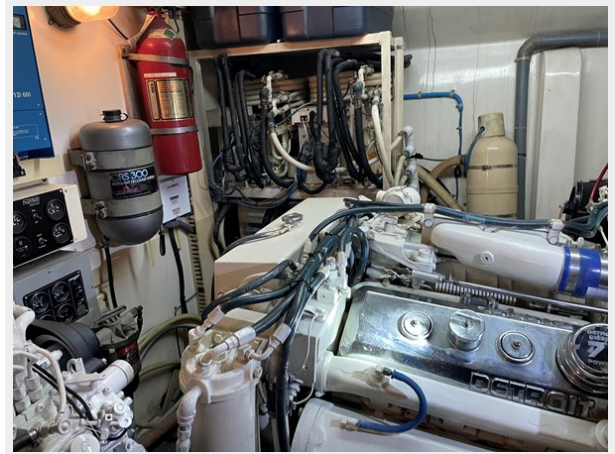
41. Engine Room view 2
