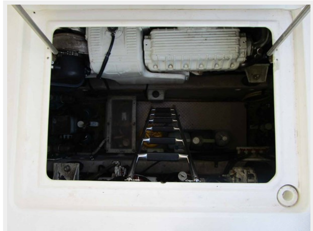
Engine Room Entrance
