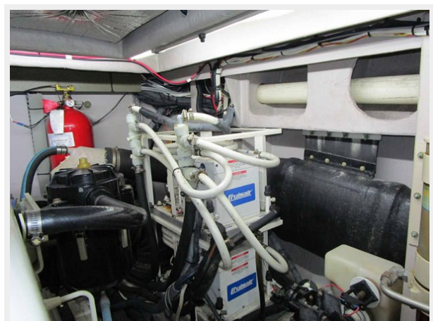
Outboard of Starboard Engine
