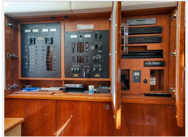
Salon Control Panel 2
