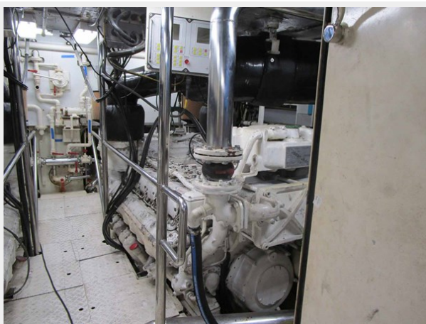
Engine Room Access
