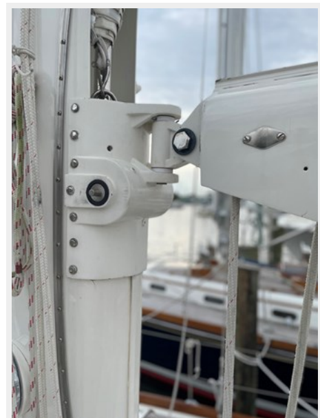
Recent Mast Paint
