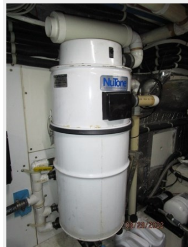
65_2787622_44_navigator_central_vacuum_system
