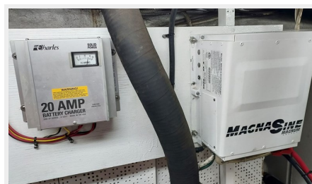
70_2787201_1099_dorcas_ann_battery_chargers_and_inverter
