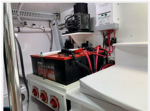
Odyssey batteries and all heavy wiring updated
