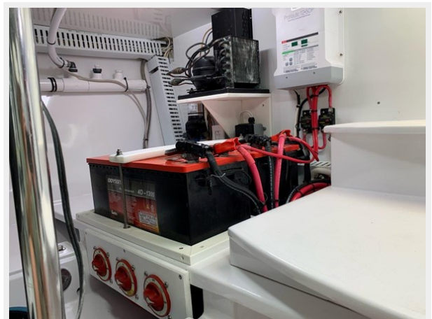
Odyssey batteries and all heavy wiring updated
