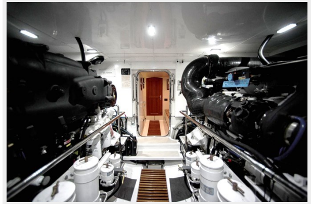
Engine Room looking aft
