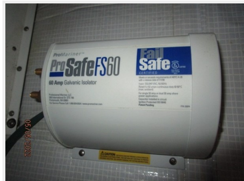
51_2788789_37_back_cove_galvanic_isolator
