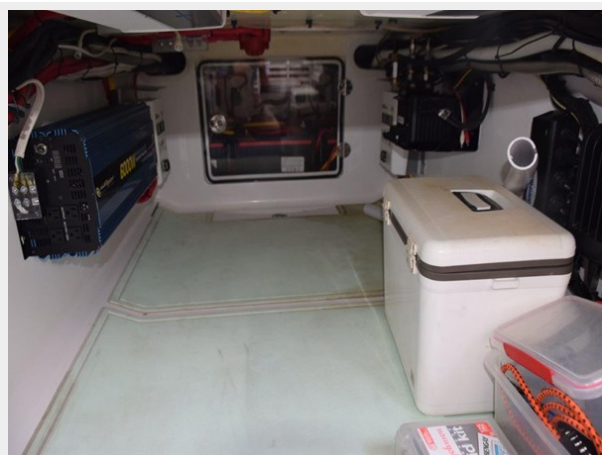
Large capacity inverter and dry storage beneath console
