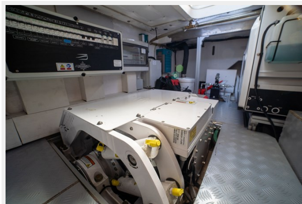
SeaKeeper Gyro Stabilizer
