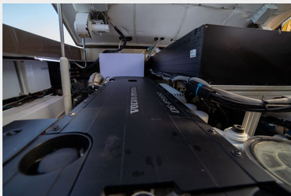
Hydraulic Lift Engine Compartment
