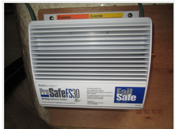
41_2789323_45_whitby_galvanic_isolator
