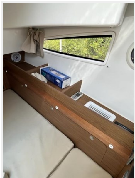
21. Mid Cabin Access to Electrical Panels.
