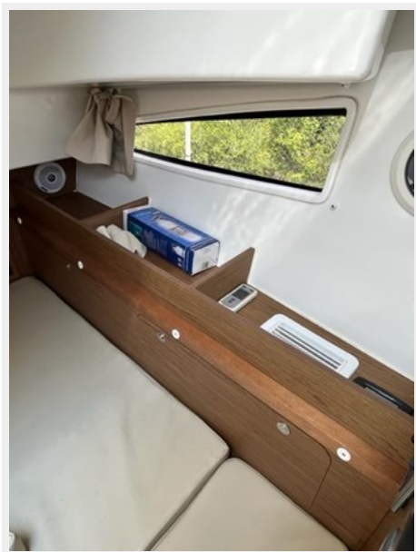
21. Mid Cabin Access to Electrical Panels.
