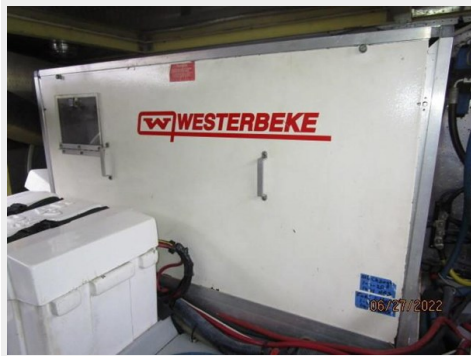
64_2790425_43_selene_generator_soundbox
