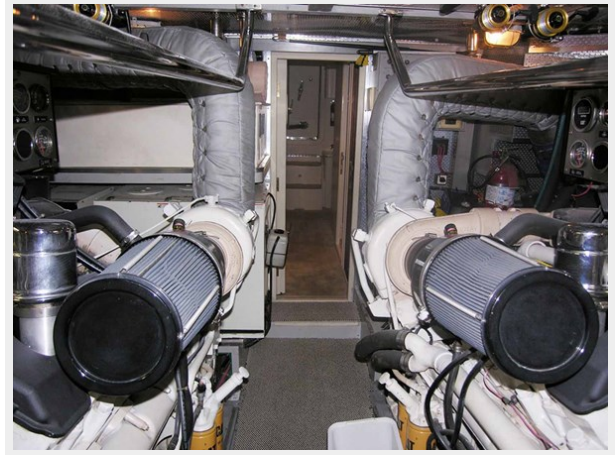
Engine Room Looking Aft
