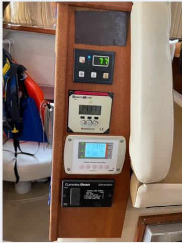
Radio Active inverter panel web1
