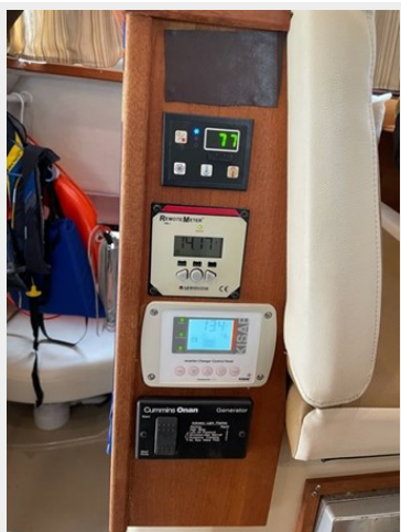
Radio Active inverter panel web1
