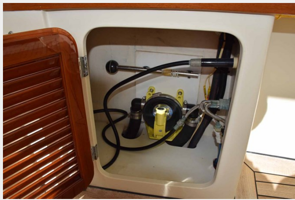
020 - Emergency hand pump
