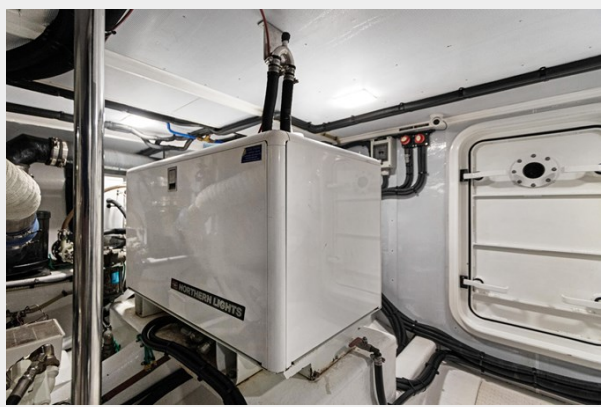
Generator stbd side
