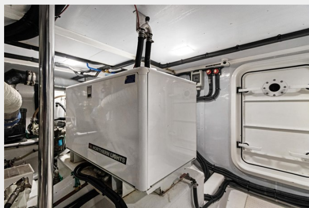
Generator stbd side
