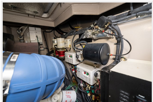
Engine room view 4
