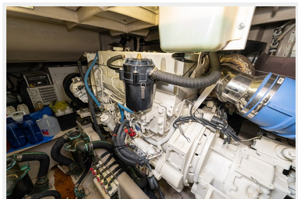
Engine room view 2
