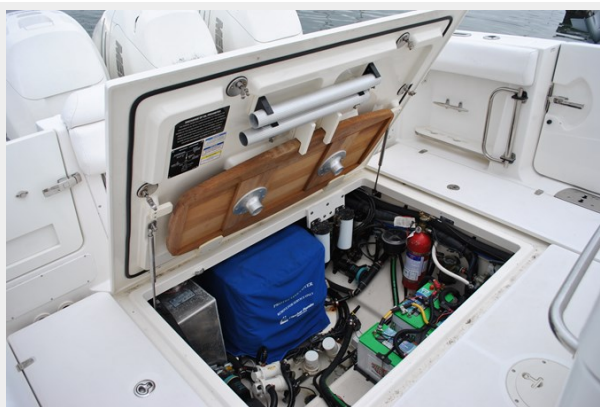
Cockpit Storage and Generator
